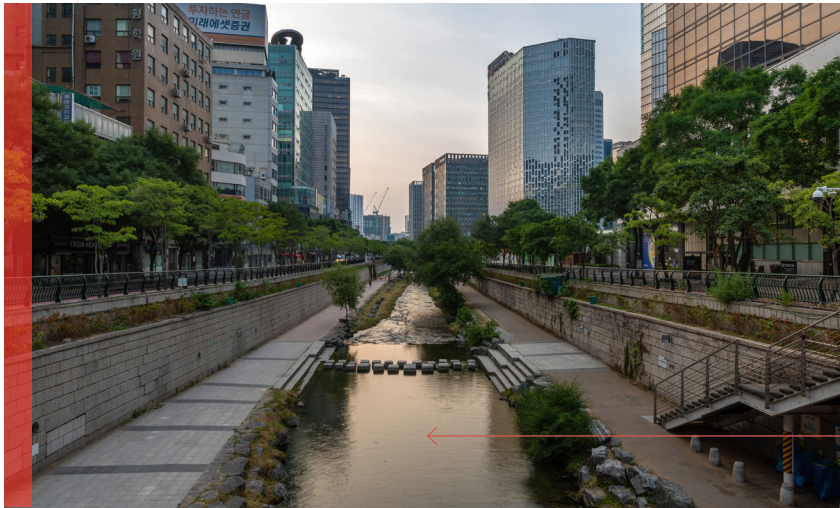
In 2005, the city of Seoul, Korea, daylighted an 11-kilometer (7-mile) stream by removing an elevated highway.
