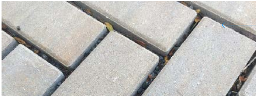
Rainwater capturing techniques: permeable pavement
