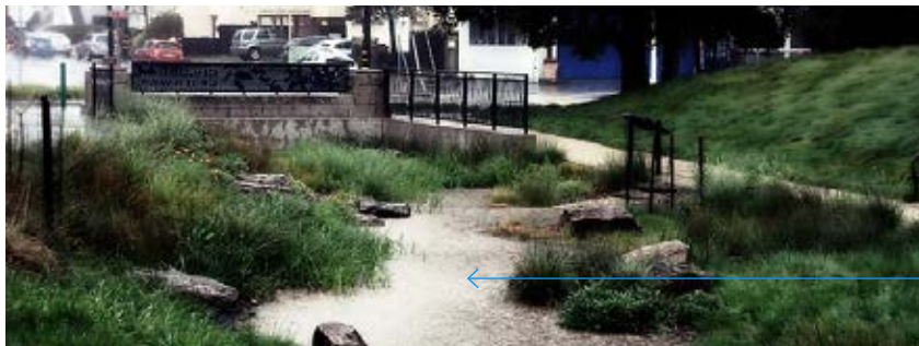
Rainwater capturing techniques: bioswale
