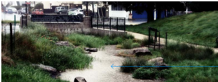
Rainwater capturing techniques: bioswale
