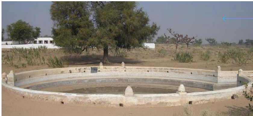
Smaller-scale water-storage projects, such as this johad in the village of Thathawata in Rajasthan, India, can have more direct benefits for locals.
