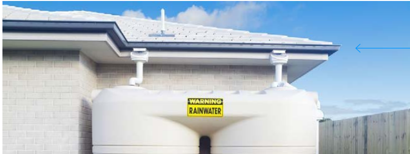
Rainwater capturing techniques: rainwater catchment system
