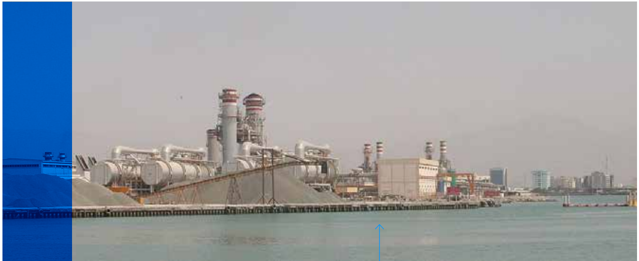
Desalination plant in Ras Al Khaimah, United Arab Emirates.
