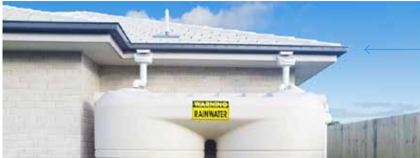
Rainwater capturing techniques: rainwater catchment system
