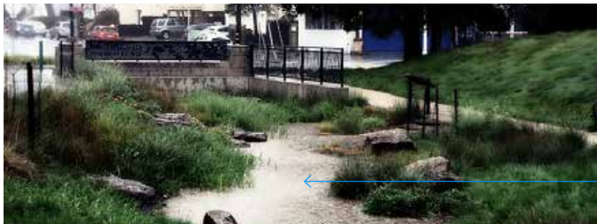
Rainwater capturing techniques: bioswale
